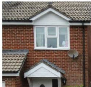
Gable front door overhang and gable wall dormer.
