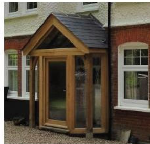
Gable portico with timber frame and glazing.
