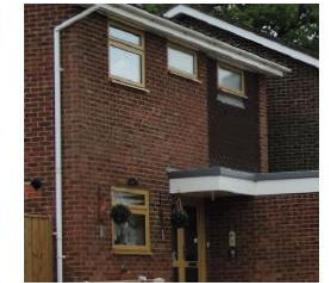
Timber framed windows and doorway.
