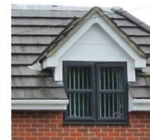
Gable dormer with painted timber casement window.
