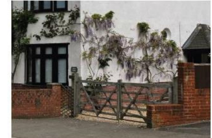
Low brick wall with timber entrance gate.
