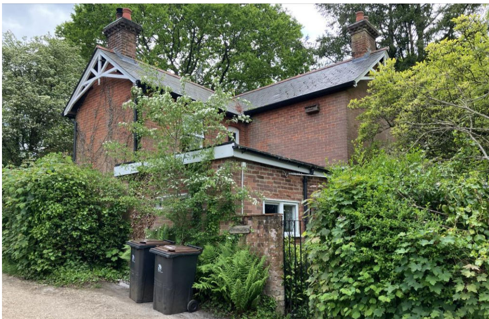
Figure 13. Decorative gable end, ridge tiles and chimneys
