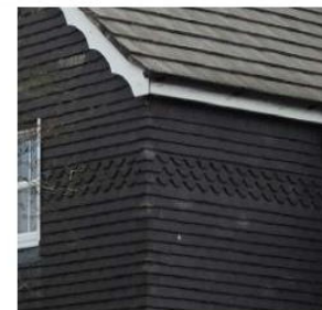
Continuous pattern in weatherboards and decorative fascias.
