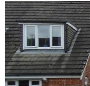
Flat roof dormer with casement windows.
